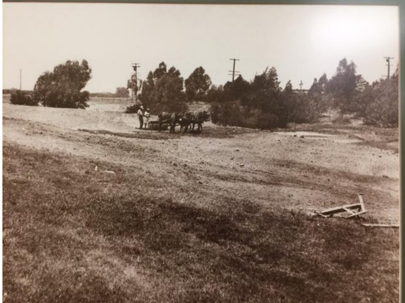
Watson's Construction crew in action
